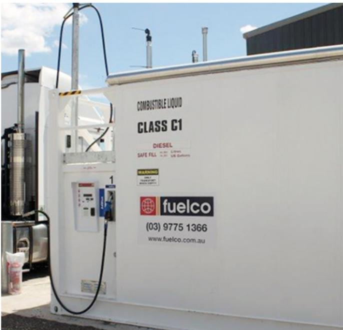
Dual Diesel and insulated DEF chemical resistant tanks
