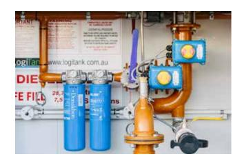
Bulk manifolds assemblies are manufactured and piped in parallel flow configurations to reduce pressure drop across the assembly and retain a high flow rate
