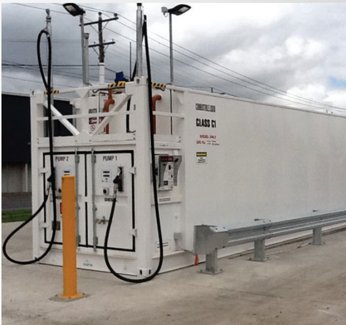
Pictured as a workshop bulk lubricant storage tank
